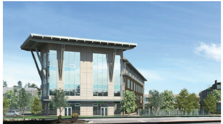
Citimark and Darwin Construction are planning to break ground by year-end 2010 at Dollarton Business Park Building C , which will include 33,973 sf of strata office space.
