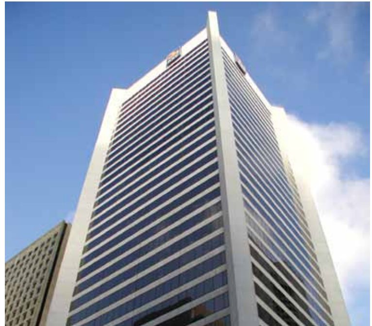
Royal Centre offers one of the largest blocks of contiguous office space in Downtown Vancouver, with 22,900 sf available
